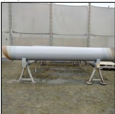
Brace ready for Installation on Lower Level
