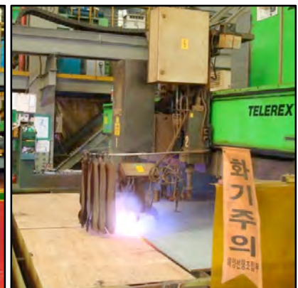
First Cut of Steel
