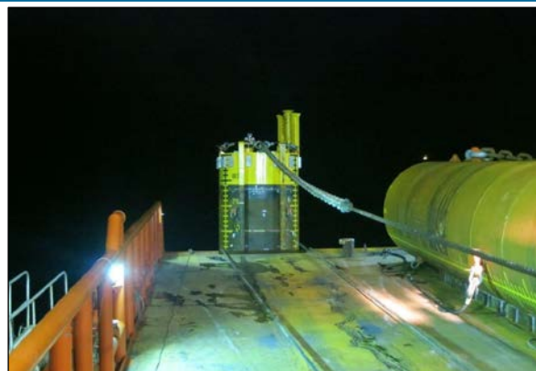
Pile Installation Going Overboard
