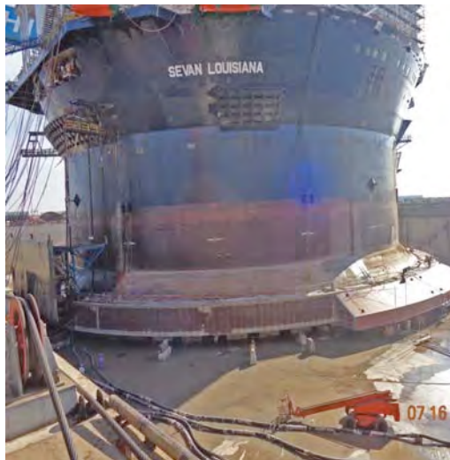
Sevan Louisiana in Dry-Dock Phase
