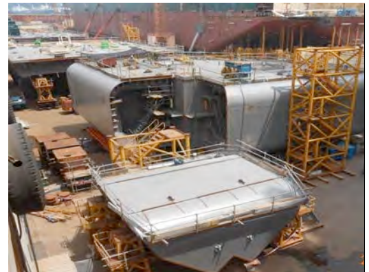
SW Node Blocks in the Dry Dock
