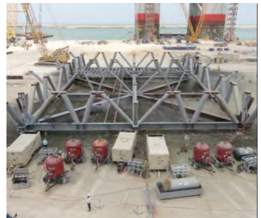
Lower Level Framing
