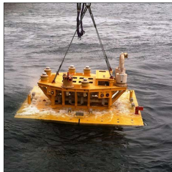
MC 253 Manifold Installation
