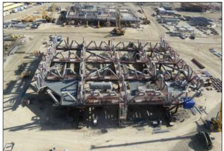
Lower Level Framing
