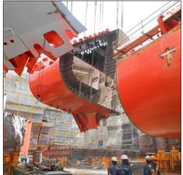
Upper Column Section Erection
