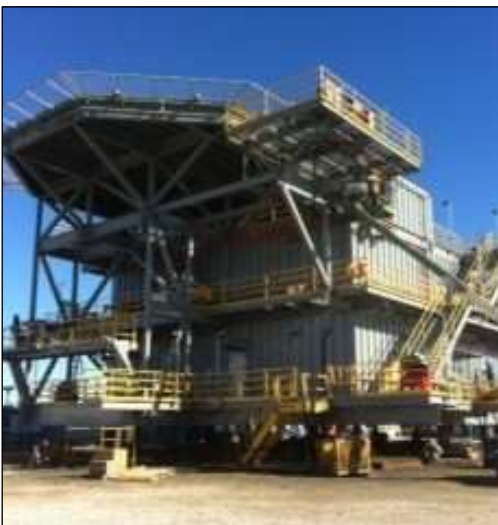
38 Man Quarters Building
