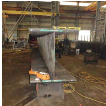
1/8—First plate girder fabricated and ready for welding
