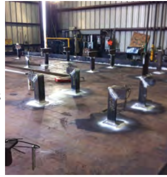
Installed Pipe Supports onto the HP & LP Flare Scrubber Skid
