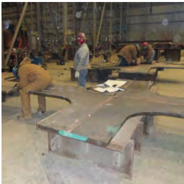
1/5—Laying out node sections to receive web plates
