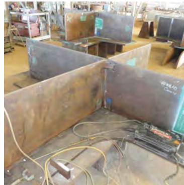
1/16—Installing web plates on node sections
