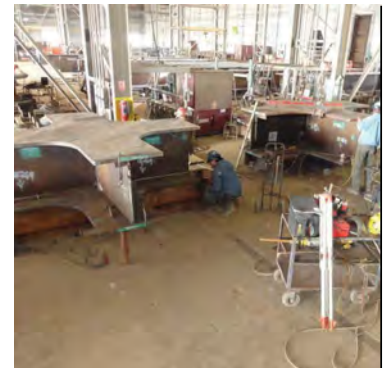
1/22—Installing final connection plate on node sections for welding
