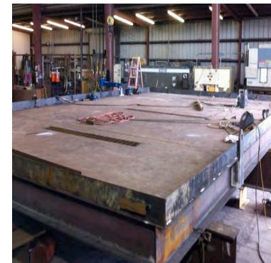
Structural skid with drain troughs, deck plate, lifting eyes & coaming installed
