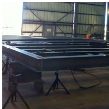
Completed Structural Skid Frame
