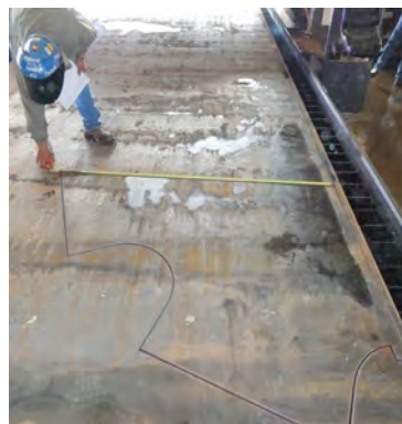
12/19—First shape cut by Kiewit
