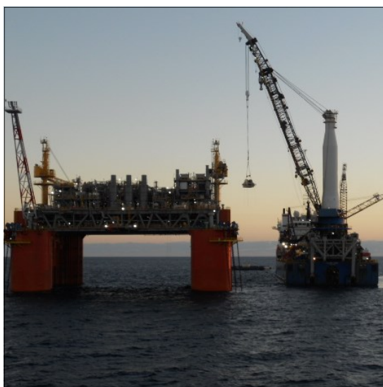
Transfer of pull-in winch from Delta House to GI200
