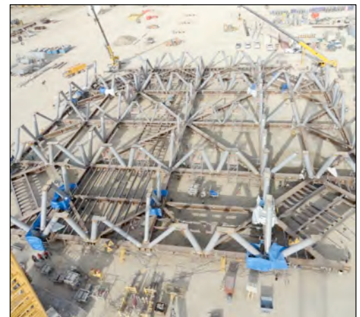
Lower Level Framing
