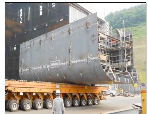
Hull Section - Southwest Pontoon Node Block (Block is on its side)
