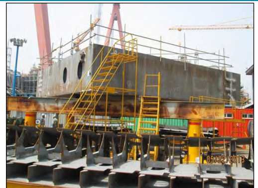
Node Section Below Potable Water Tank
