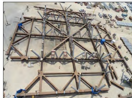
Lower Level Framing
