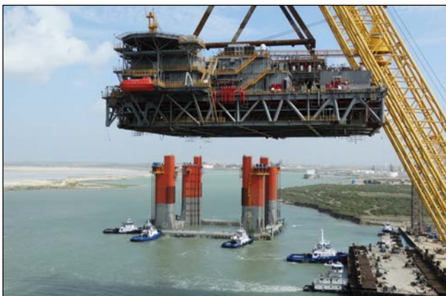
Lifting the Deck
