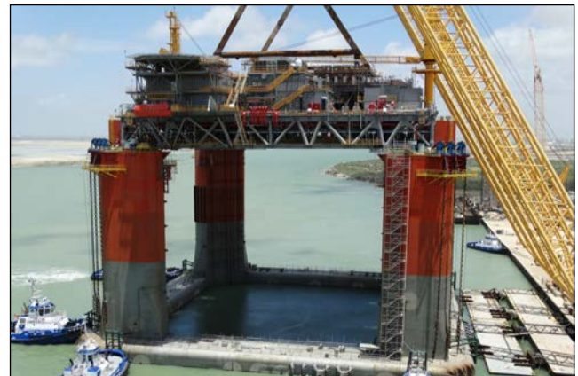
Setting of Deck on the Hull
