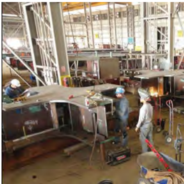
1/29—Lower level node sections in progress in various stages
