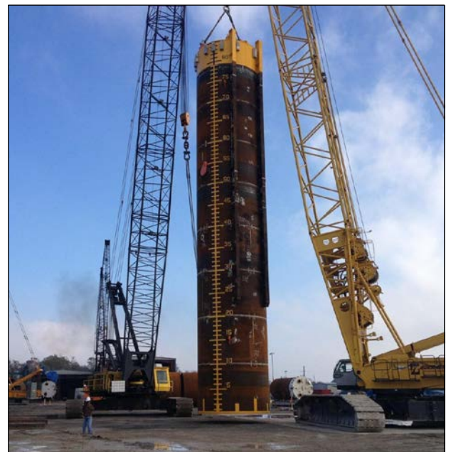
Pile 1 Lift Test
