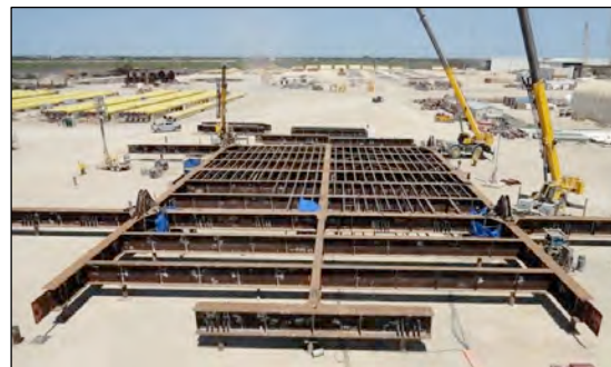
Upper Level Framing
