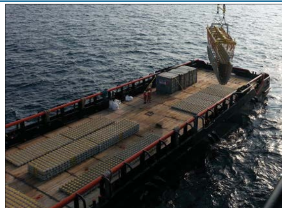
Concrete Mat installation
