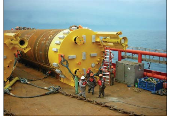
Pile on deck of the M/V Joshua Chouest
